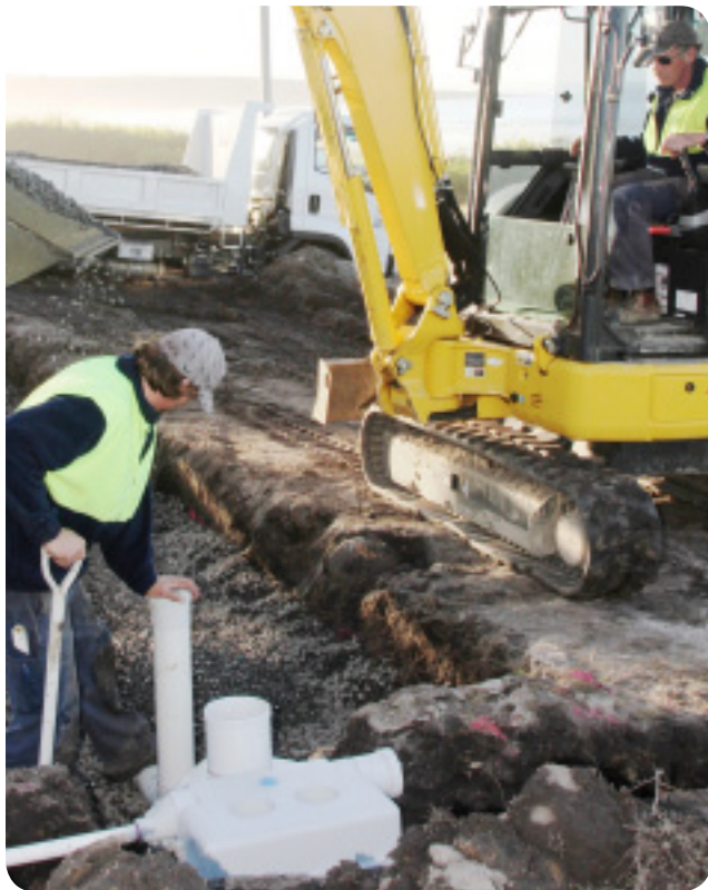
A typical evapo-transpiration bed under construction.
