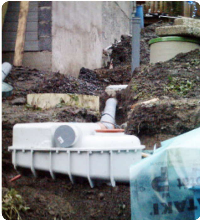
Installation at the head of evapo-transpiration bed for even waste water distribution.
